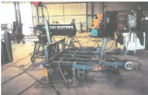
Main frame Construction
